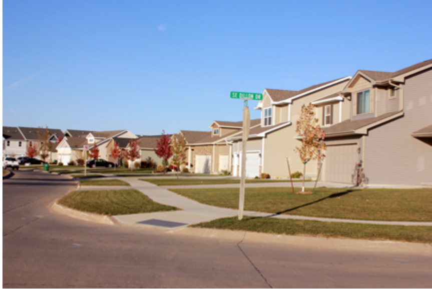
Figure 25: A typical street in Glynn Village looks similar to the conventional suburban street. The garages front the street, and many houses have similar architectural form and details, if not the exact same house plan only mirrored.
